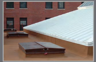
ROOF HATCH + SMOKE VENT
