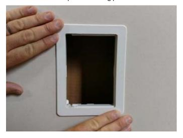
2. Remove door from frame and apply adhesive to backside of flange.
